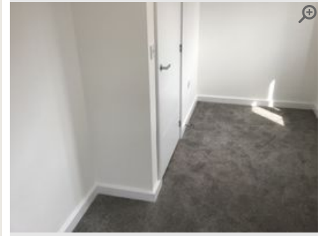
Provided by Inspector Captured (via App): 27/08/2024 12:35 PM Added 27/08/2024 Reference 6.1.3
