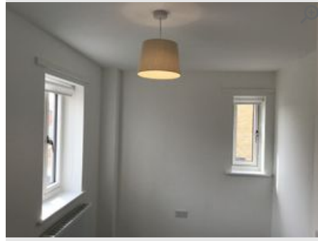
Provided by Inspector Captured (via App): 27/08/2024 12:35 PM Added 27/08/2024 Reference 6.1.2
