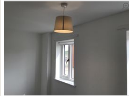
Provided by Inspector Captured (via App): 27/08/2024 12:35 PM Added 27/08/2024 Reference 6.1.6
