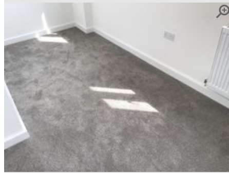
Provided by Inspector Captured (via App): 27/08/2024 12:35 PM Added 27/08/2024 Reference 6.1.5
